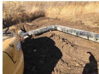
4. Header tie-in to existing system
