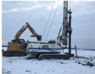
3. Drilling well through vacuum box to reduce odors
