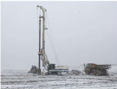
1. Speciality gas drilling rig mobilized to well site
