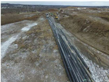
1. Header pipe welding
