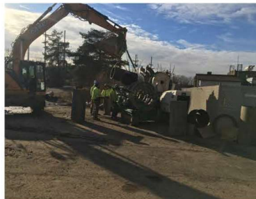
3. Fusion welding at gas to energy plant/flare
