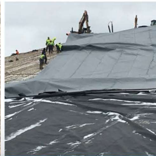
Deployment of geomembrane cover
