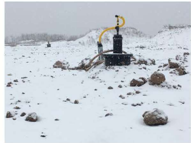
4. Completed gas collection well
