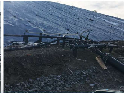
Completed geomembrane cover with gas collection
